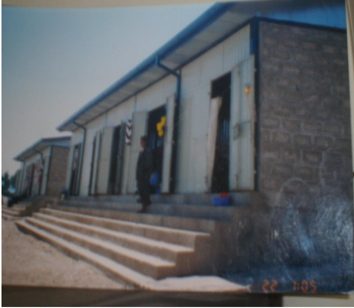
Market Stall constructed by WISE
